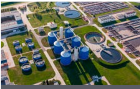
Sewage treatment plants
