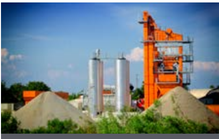
Asphalt mixing plants
